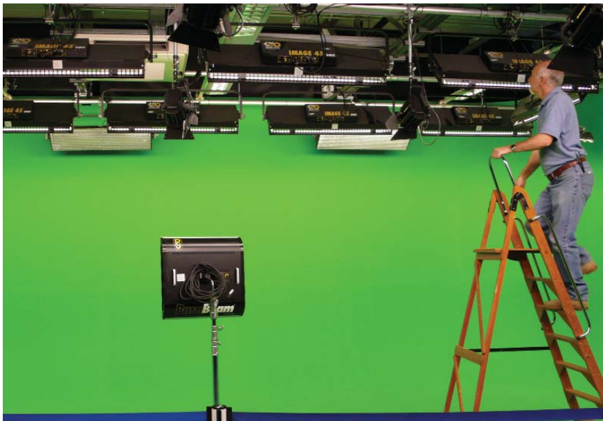
20' x 20' (7m x 7m) visual effects green cyc and floor lighted from above with Kino Flo Image fixtures, lamped with True Match® 3200K full spectrum tubes.
